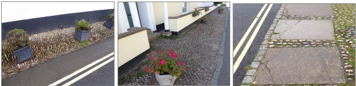
Photos: Examples of hard surfaces, showing how original cobbles and granite setts have maintained a better condition than the replacement concrete surface
